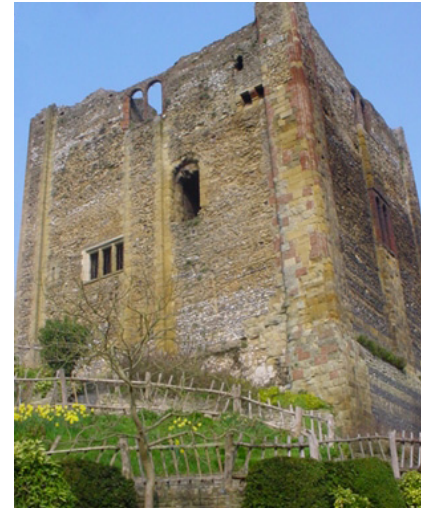
View of keep prior to conservation work
